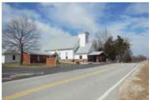
51 Cyntheanne Road south and west elevations
