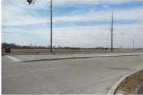
Street at Cumberland Road looking west
