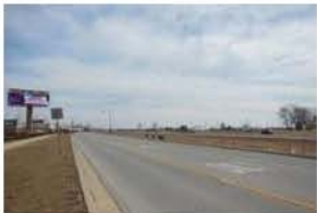
1st Street at Norell Road looking north
