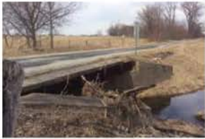
Bridge Deck at Thorpe Cree
