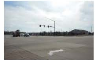
Street at Cumberland Road looking south
