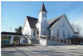
1425 Lantern Road east and north elevations
