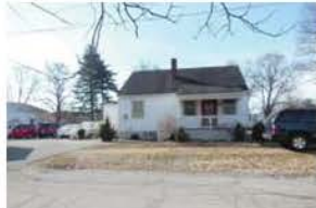
oad_11478 Lantern Road Ne
