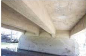
177_underside of deck N span
