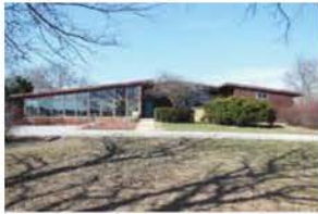
SR 13 SR 13_front elevation_loc
