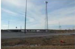
Looking SE to I-69 from 1165t
