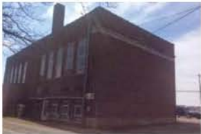
015 8791 W 800 S north and east elevations
