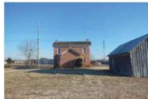
106th Street House south elevation
