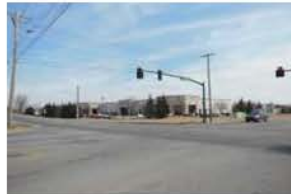
Street at Cumberland Road looking west
