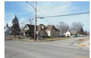
479 Lantern Road east and north elevations
